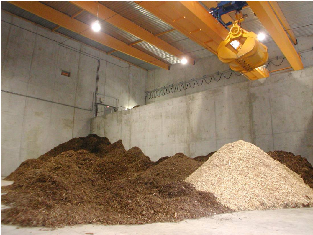
Chaufferie bois Venissieux (C) ALE
